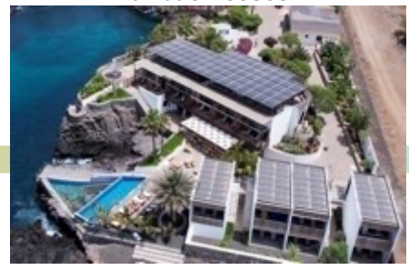
Clean water from solar energy for businesses
